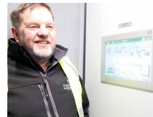
Richard Norris next to touch panel interface controlling and regulating power output
