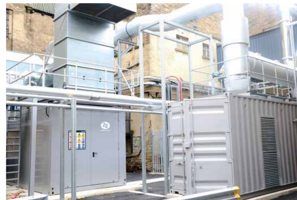
Curtis发电厂减小碳足印
